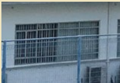
Inner façade: Original steel windows have been replaced with aluminum casement windows.
