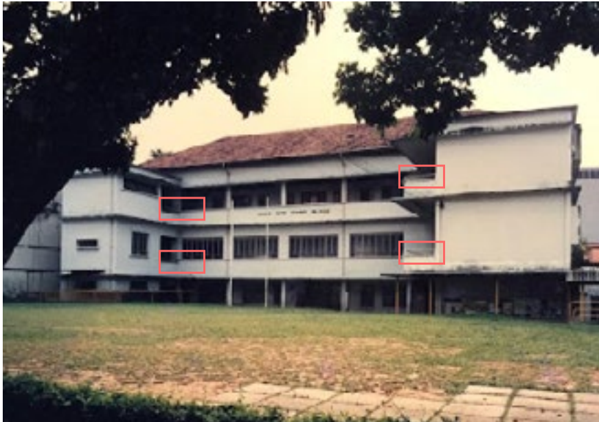
Archive: Decorative mild steel railing, coupled with a lower parapet, breaks the mass of the solid building form.
