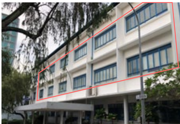
Emerald Hill Road façade – Present
