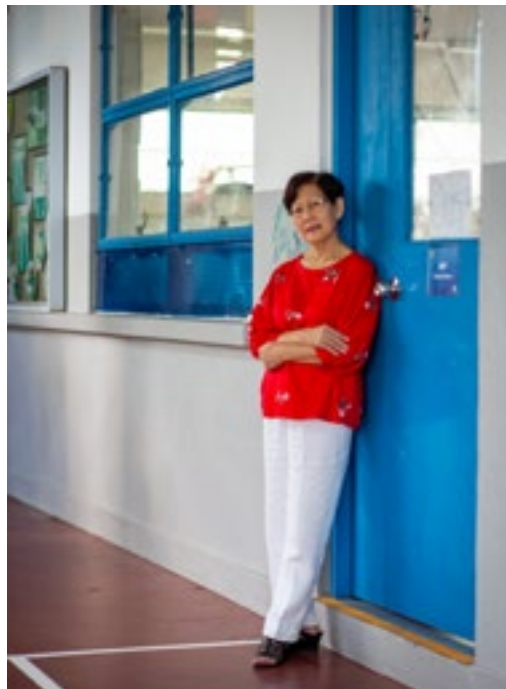
Present: The elegantly framed steel window stands in stark contrast with the oddly proportioned timber door that was a latter day addition.
