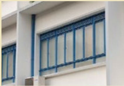
Emerald Hill Road façade: The original steel windows appear to be intact.
