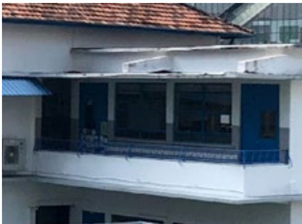
Present: Original decorative mild steel railings can still be found on site today.
