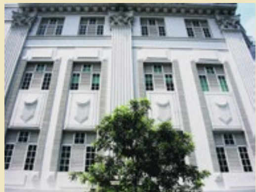
The Loke Yew Building in distinctive Art Deco style was designed by E.C. Seah in 1931. 17
